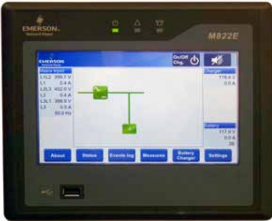
Chloride CP-70RC - Local human-machine interface (HMI)
